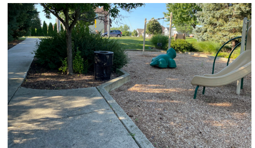
High curb and no ADA ramp
