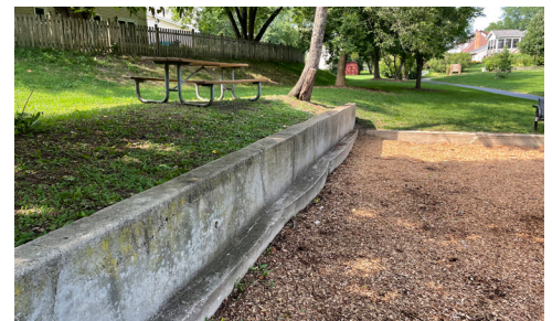
Playground retaining wall
