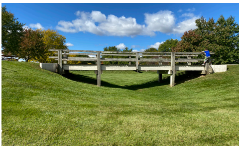
Detention basin / pedestrian bridge
