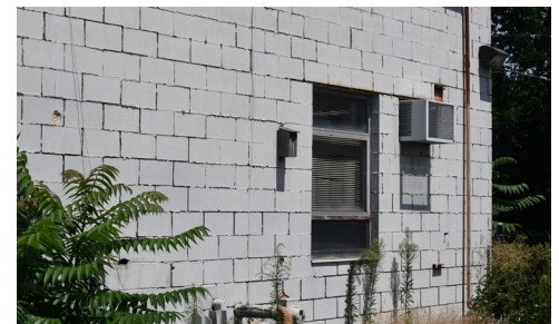
Tuck-pointing and windows
